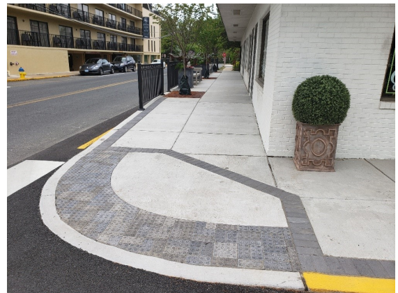
ADA Compliant Sidewalk at 2nd and Baltimore
